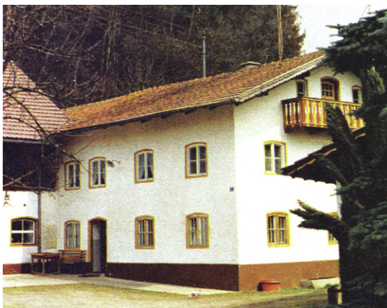
Fig. 7-36 This house in the Bavarian forest near Munich derives its electric power from a small generator, powered by water from a canal.
